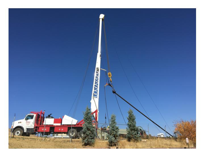
Pictured above, the District's operator (Colorado Water Systems) and several utility contractors are working on one of the District's many water wells. Each fall, the Stonegate Village Metropolitan District conducts repairs and maintenance, usually overhauling at least one of the District's deep Denver Basin Aquifer groundwater wells. The water wells are the backbone of our municipal water supply, and the
