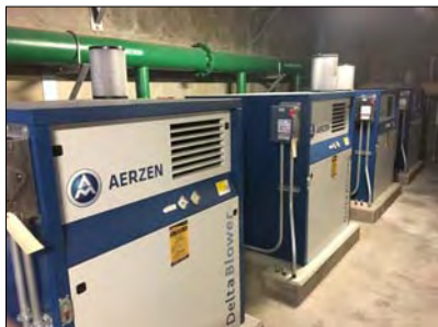
Blowers that aerate the Waste Water Basins
