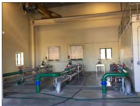
Blowers that aerate the Waste Water Basins
