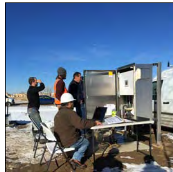
SCADA Programmer Setting Up WISE System Radio Telemetry
